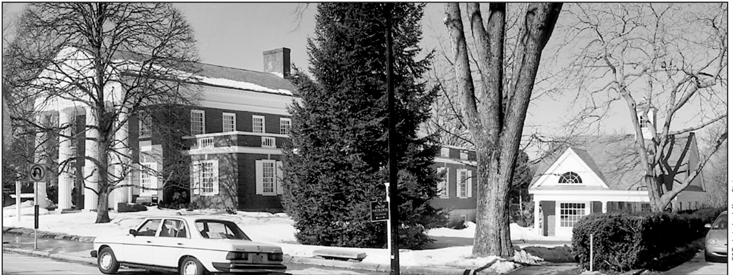
The Concord Visitors' Center, located at 58 Main St. in Concord, was designed by Nashawtuc Architects, a firm located in the same community.
